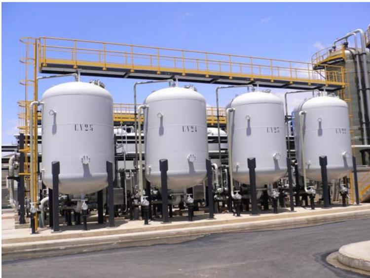
Figure 2: Water treatment plant with GFH used in four parallel filter containers, designed to treat 4,000  $\text{m}^2$  of water daily like that from the reservoir lake in the Olympic Park in Beijing.
